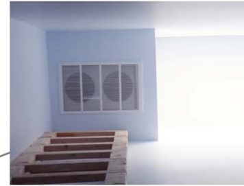
Whole house fan at top of clerestory withdraws heat from the house and provides ventilation.
