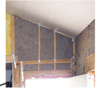
Cellulose insulation made from recycled newsprint., providing minimal air infiltration and a high R-value.
